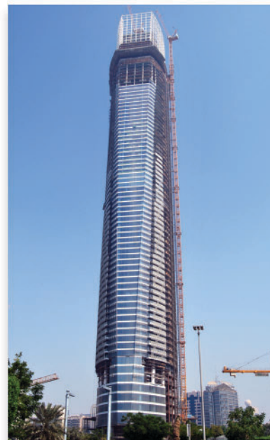
Landmark Tower in Abu Dhabi featuring BLÜCHER stainless steel drains
