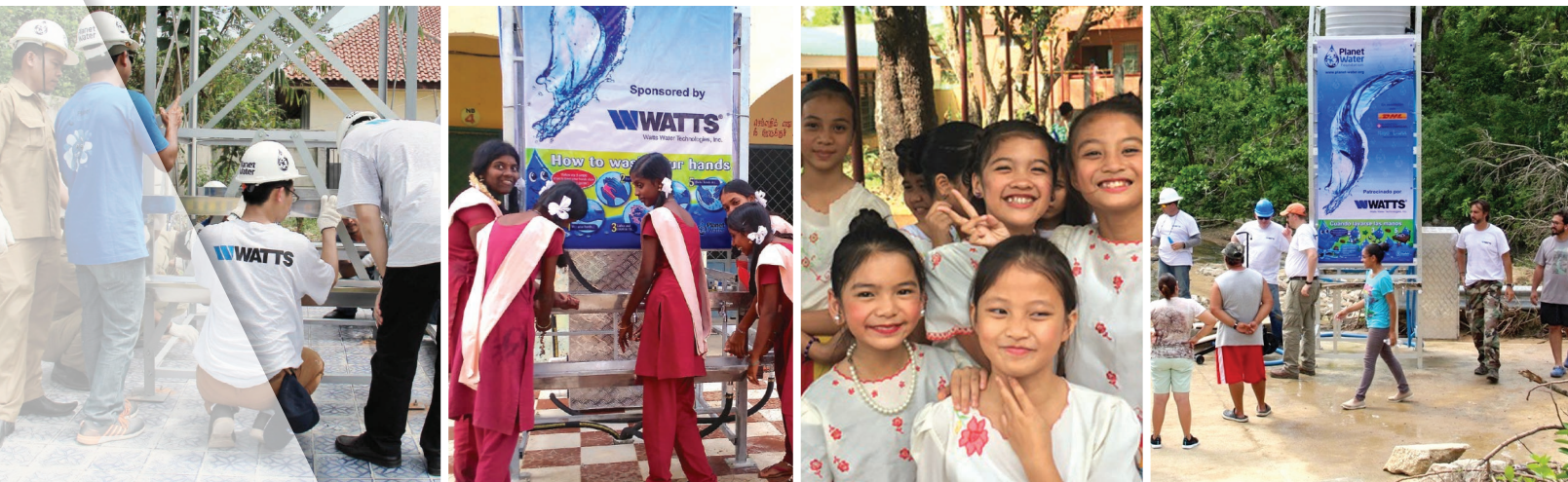
Installing AquaTowers in (left to right) Indonesia, India, the Philippines, and Puerto Rico.
