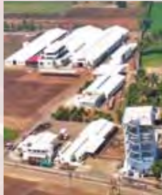
BG Chitale facility
