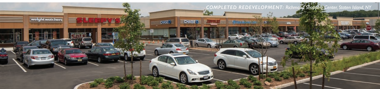
REDEVELOPMENT IN PROGRESS: Cupertino Village, Cupertino, CA
