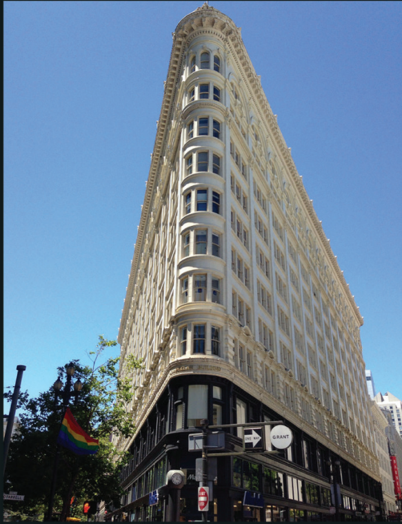
PHELAN BUILDING, SAN FRANCISCO, CA
