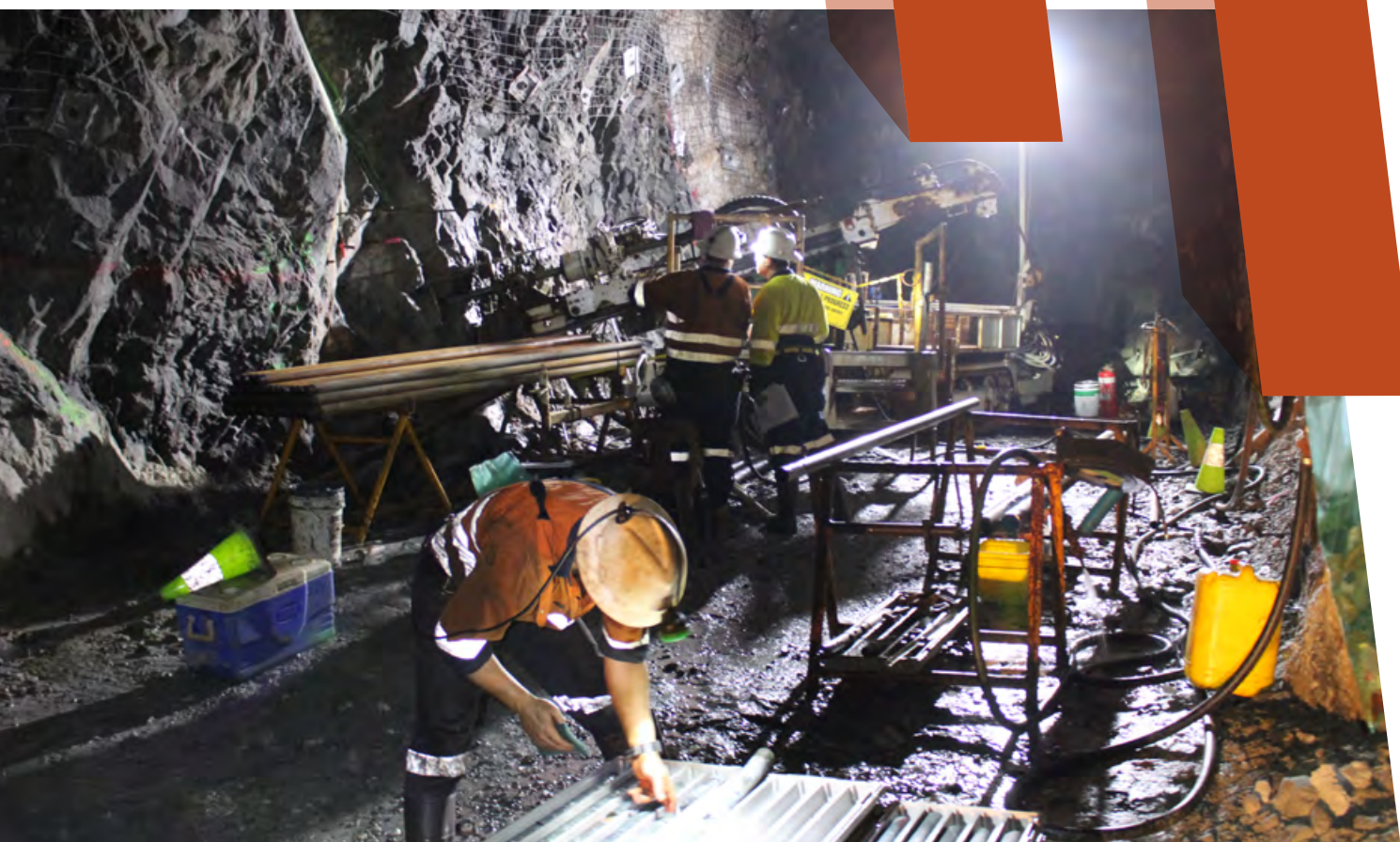
Figure 4: Underground drilling in progress
