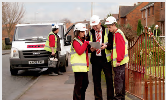
Repairs and maintenance, Lambeth
