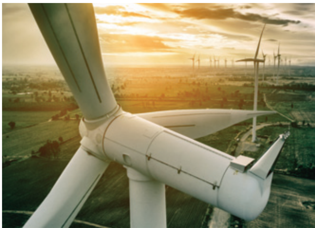
Emerging industries like wind and solar rely on Iridium's real-time telemetry and sensory data to monitor remote infrastructure and efficiently route power across the globe with minimal loss. This connectivity also supports timely maintenance and safety for lone workers that service these alternative energy assets, many in remote areas.
