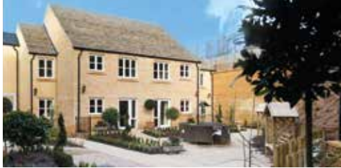
Saxon Grange, Chipping Campden
