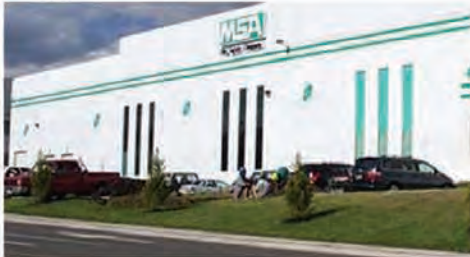
MSA's new 77,000 sq. ft. manufacturing facility in Querétaro, Mexico opened in December, marking MSA's 50th year of doing business in Mexico.
