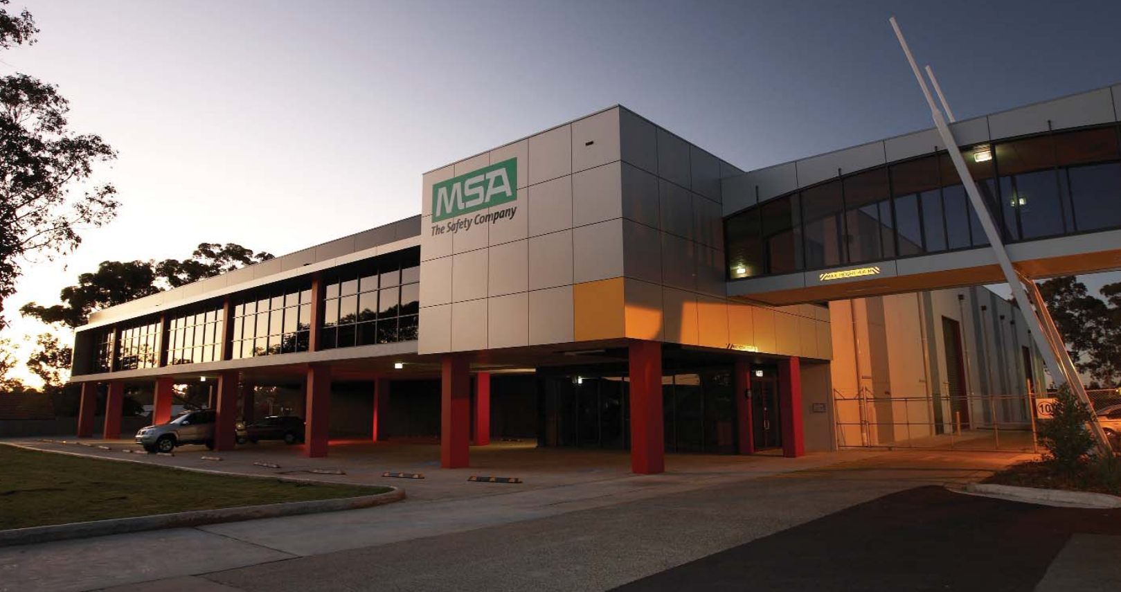
The conversion to DFT is already underway at some of our international manufacturing facilities, including Australia. Shown above is MSA's office in Sydney.
