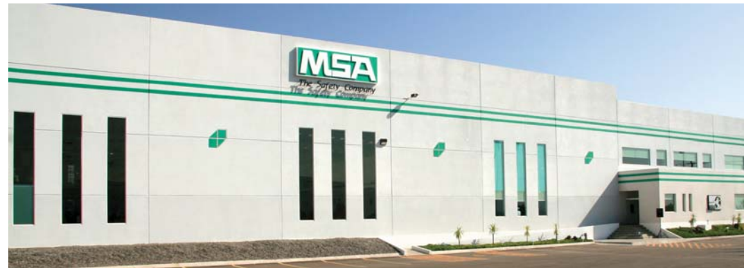
Marking 50 years of doing business in Mexico, MSA opened its 77,000 sq. ft. facility in Querétaro at the end of 2007.
