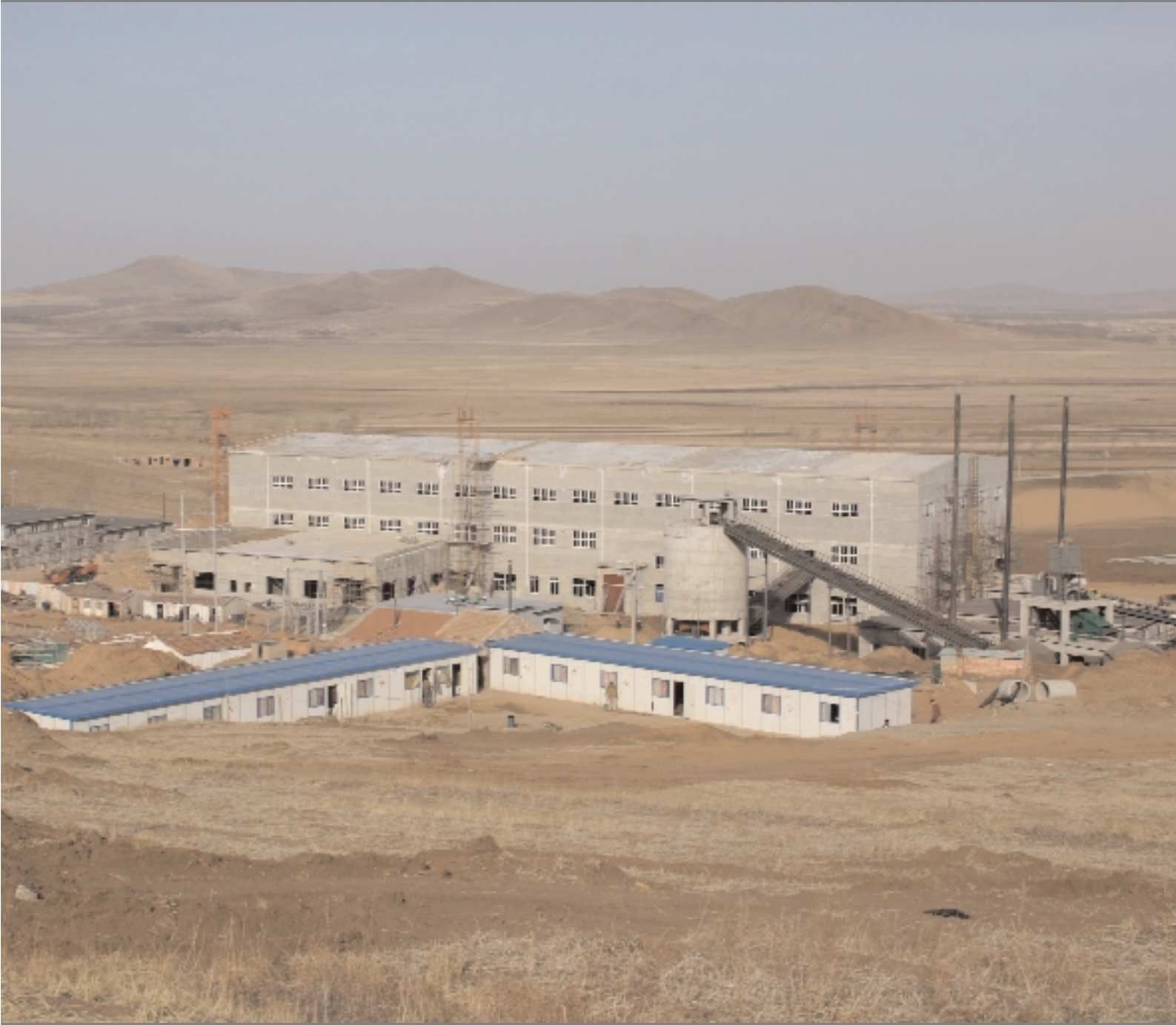
The processing plant at Caijiaying
