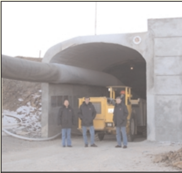
Main production portal
