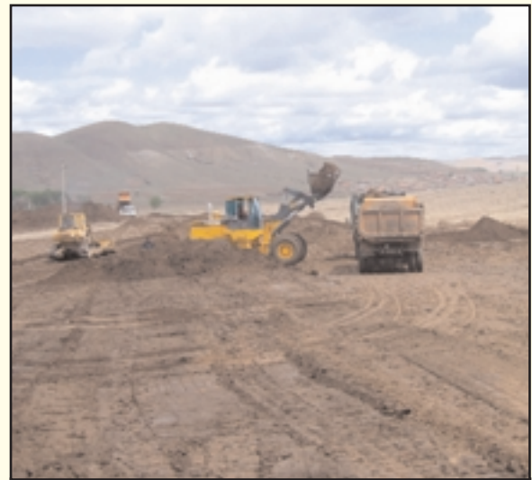
Processing plant site preparation May 2004
