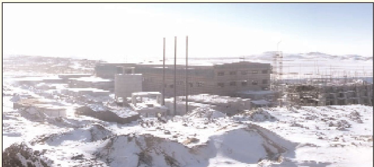
Panorama of Caijiaying processing plant during construction in the winter
