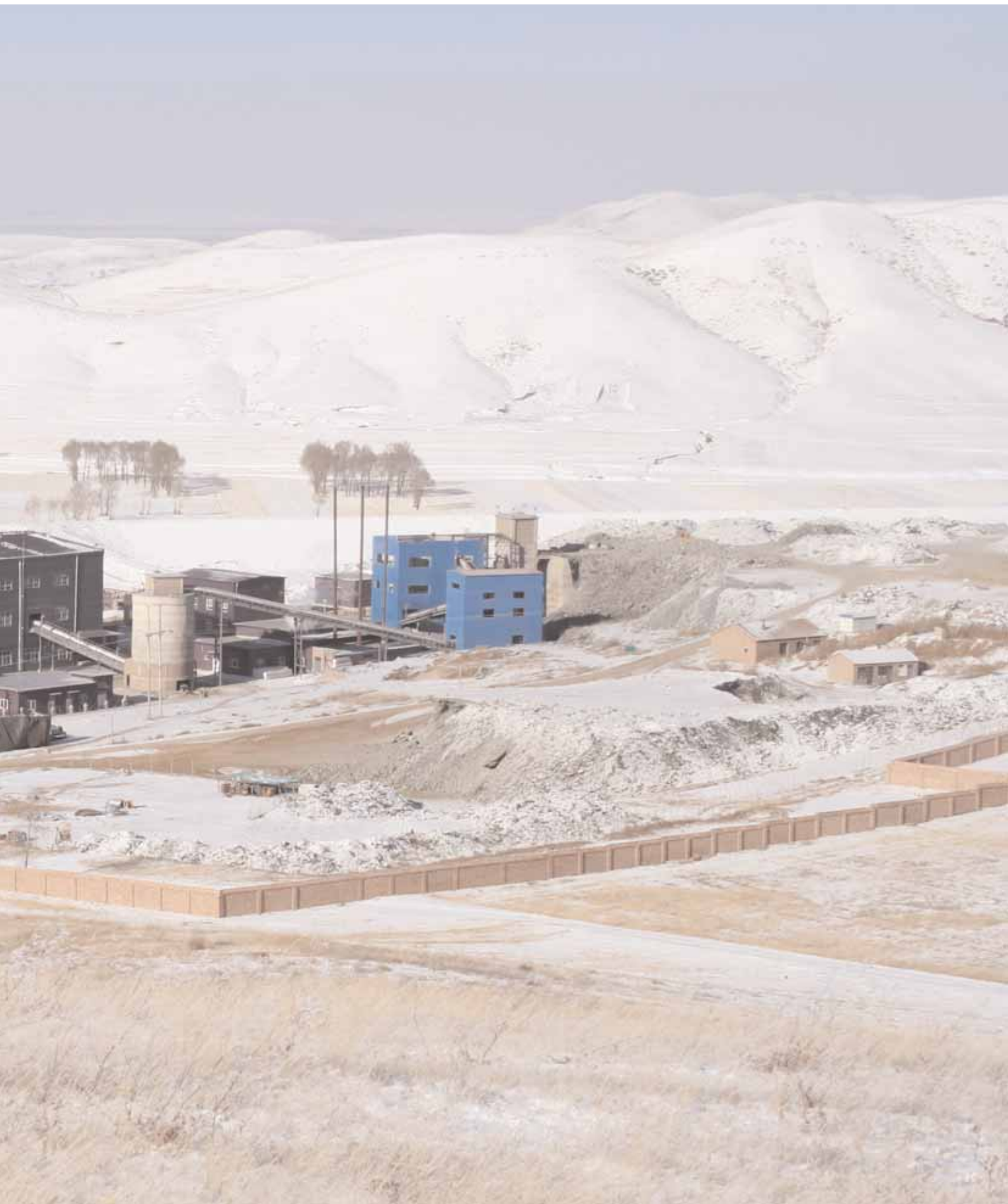
CAIJIAYING PLANT WINTER 2006
