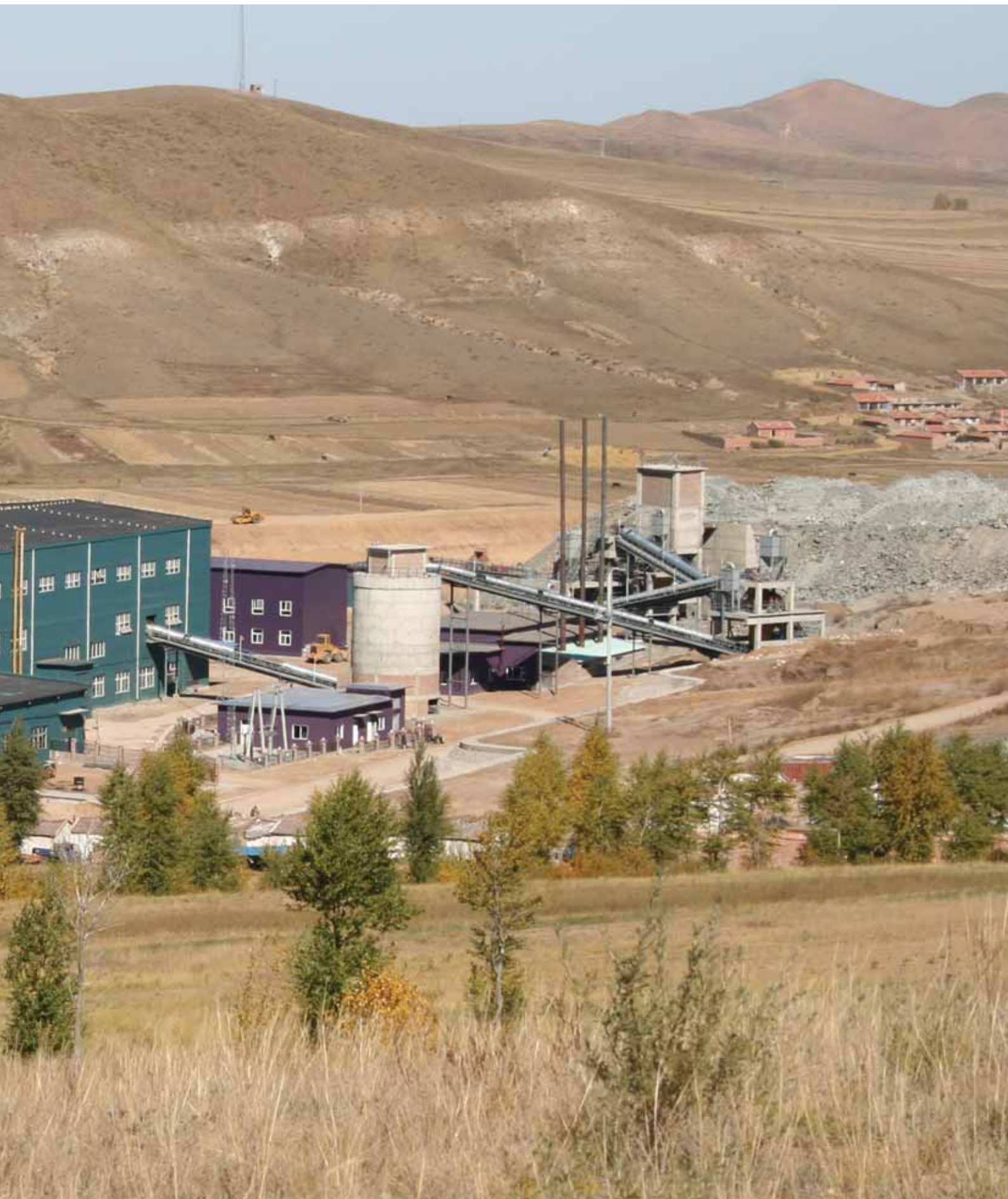
CAIJIAYING PROCESSING PLANT AUTUMN 2005
