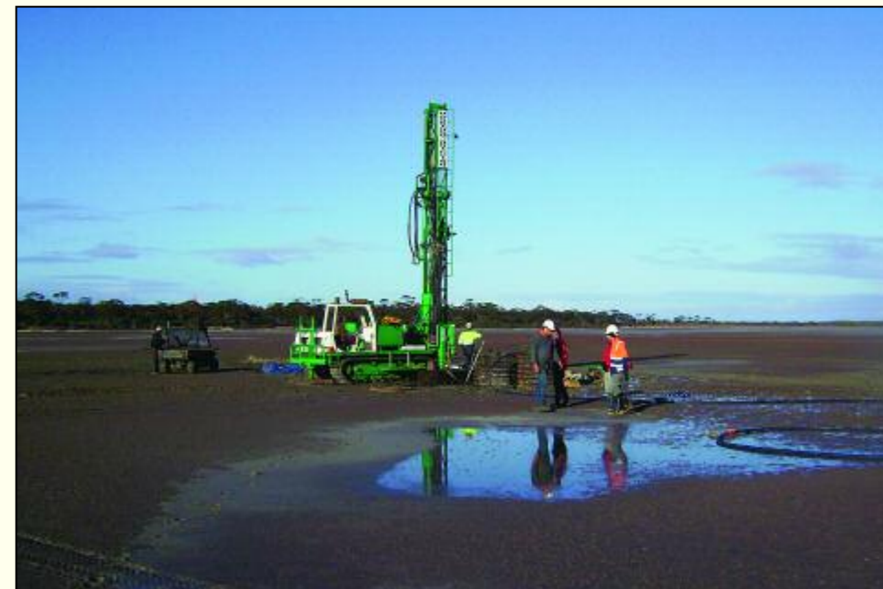
Drill Rig at Salmon Gums
