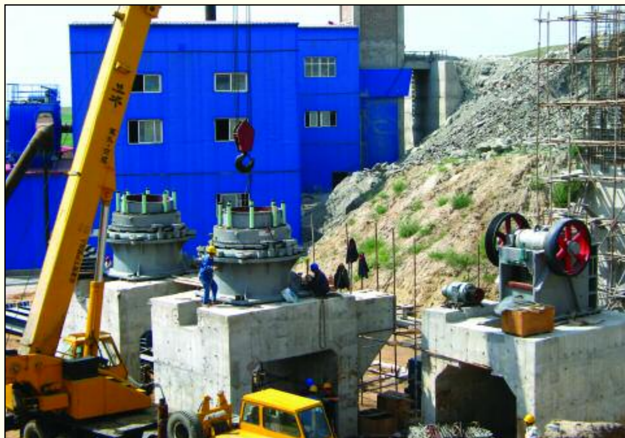
Caijiaying Mine Site - Plant Upgrade Construction
