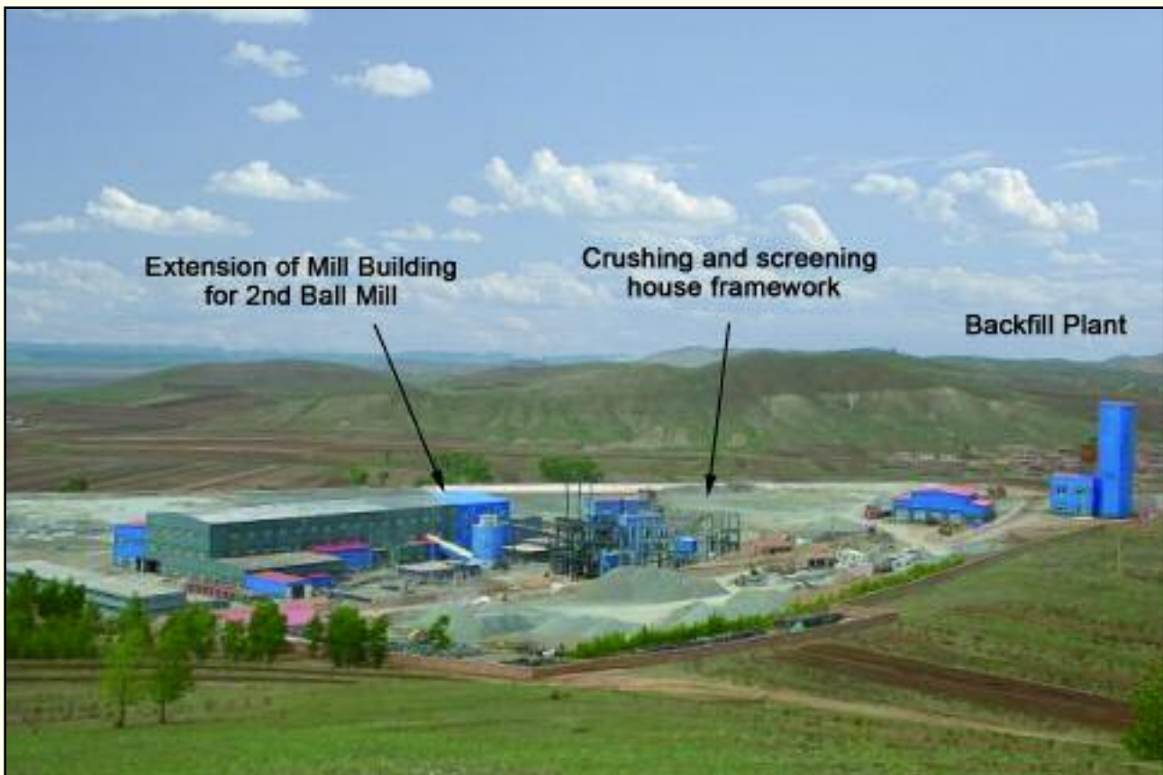
Caijiaying Mine Site Showing New Structures
