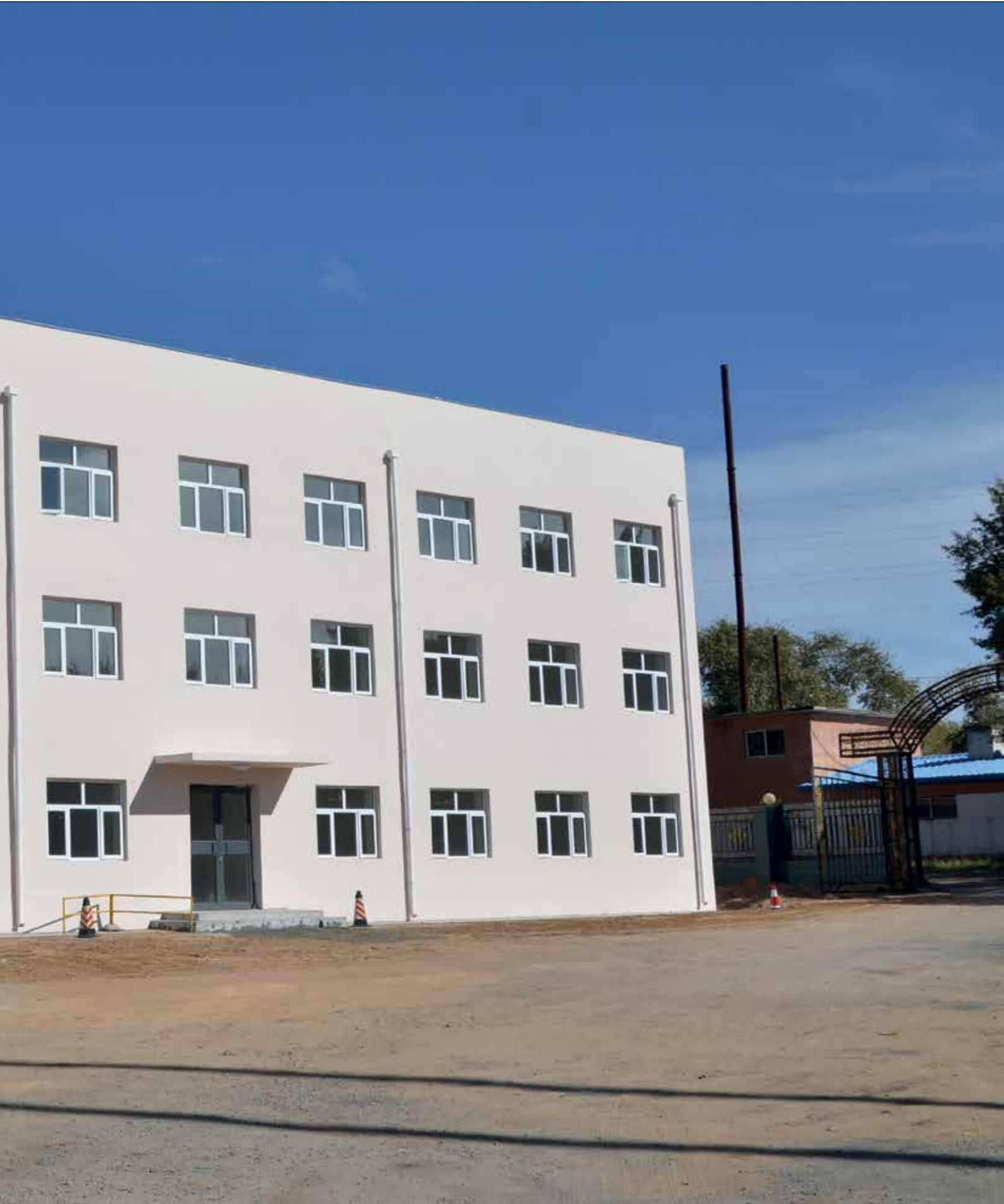
New accommodation block for Chinese personnel at the Caijiaying Mine camp site 27
