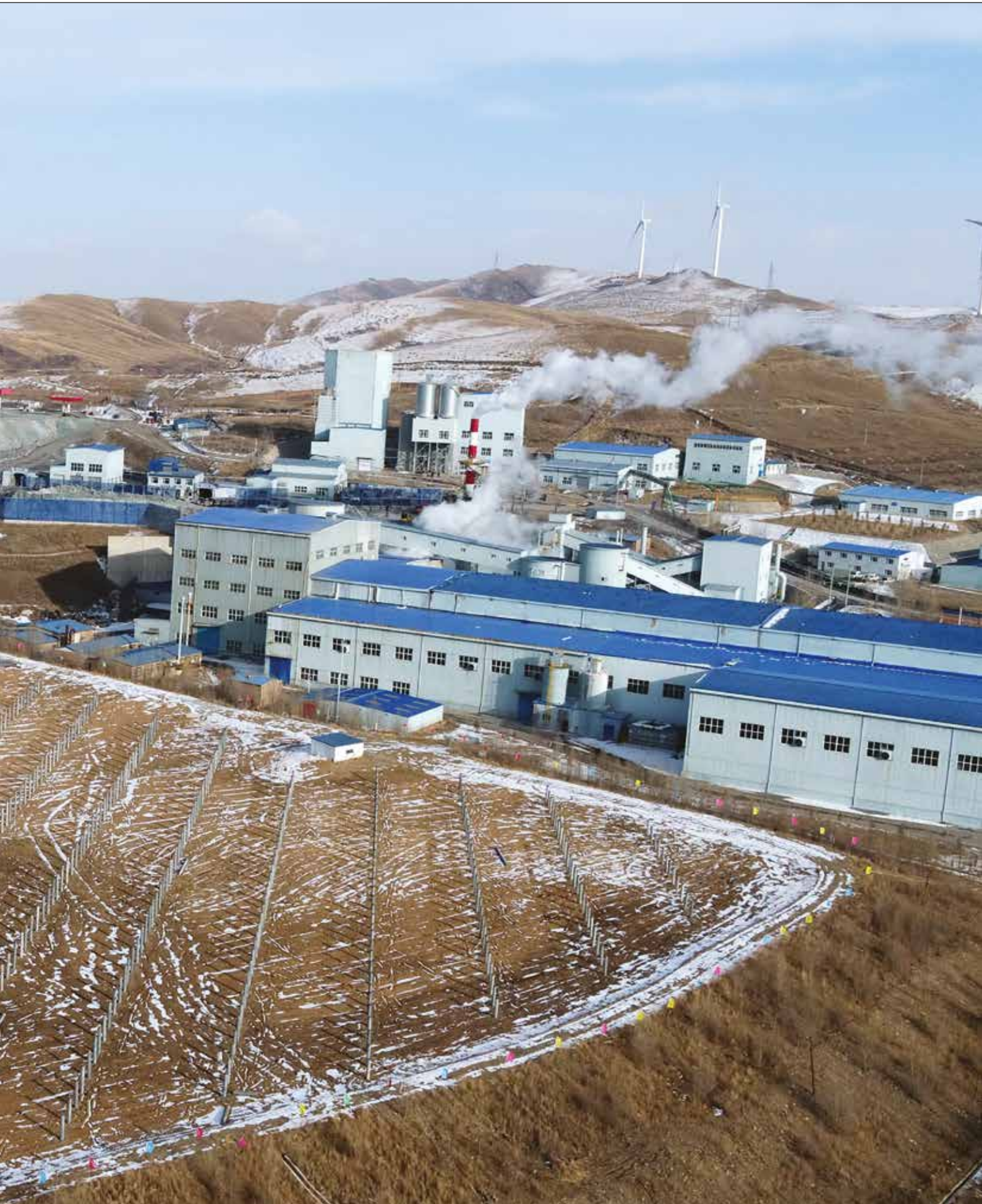
Rehabilitated tailings facilities 1 and 2 with foundations and posts awaiting installation of solar panels for generation of solar power for the Caijiaying Mine.
