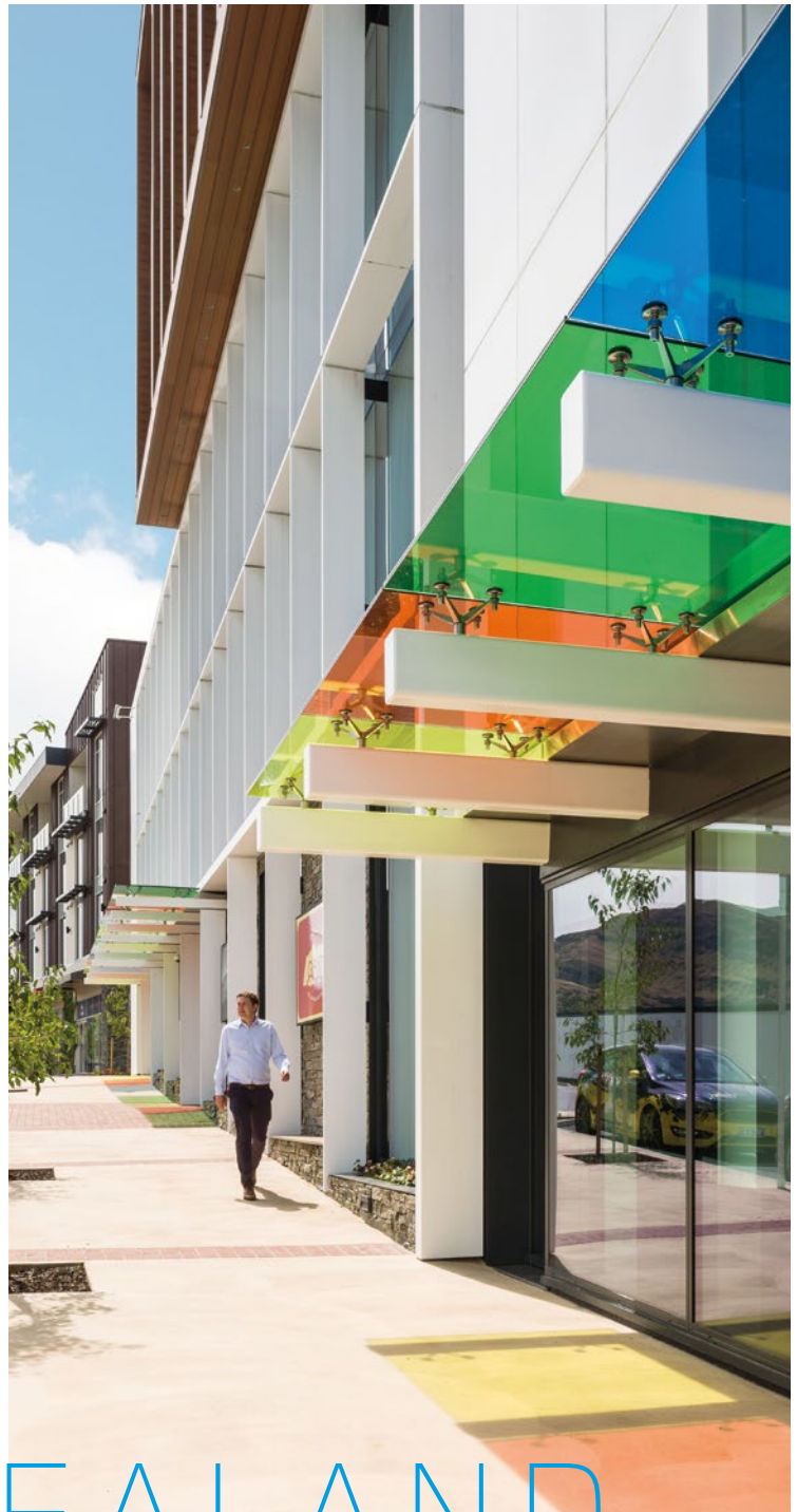
Hotel Canopy Laminated Toughened Safety Glass with PET Coloured Films.
