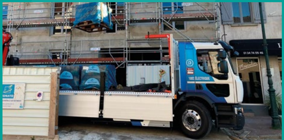
One of our electric trucks on site in France
