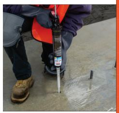
In July, we expanded our line of concrete products with our **AT-3G™** all-weather hybrid-acrylic anchoring adhesive. It's engineered to deliver a faster-curing, high-strength bond for cracked and uncracked concrete.
