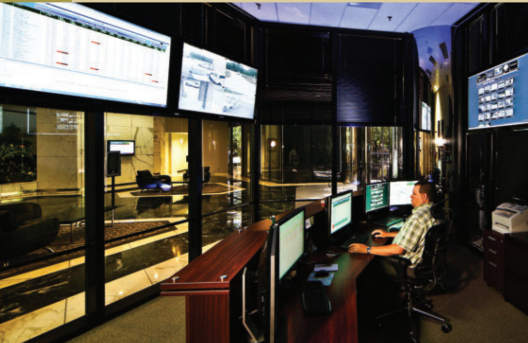
EXCO's Field Operations Control Center
