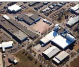
Engineered Films' manufacturing campus expanded in fiscal 2007 as this group increased its extrusion capacity by 60% to 80 million pounds a year.
