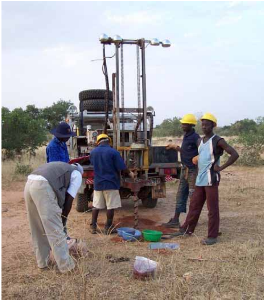
Power auger drilling on Laterite Hill Grid
