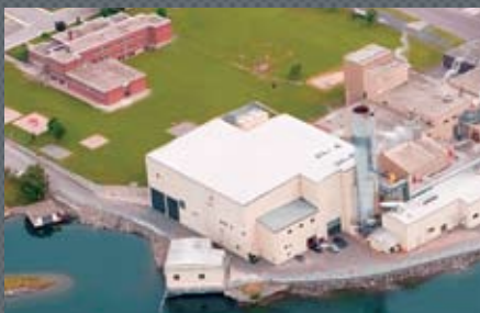
Cardinal provides the adjacent Benson Public School with free heat.
