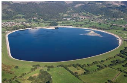
Providing safe water systems is a crucial and growing part of infrastructure demand around the world.
