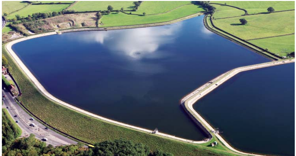
Bristol Water provides 240 million litres of water every day to a local population of 1.2 million.
