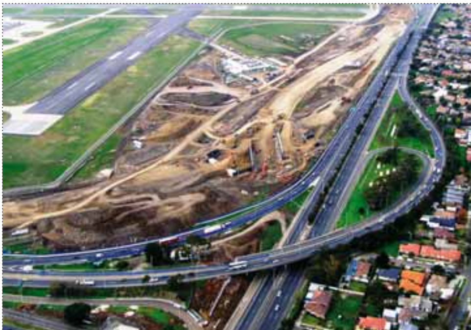
< Works continue on the $150 million upgrade to the Tullamarine-Calder interchange.
