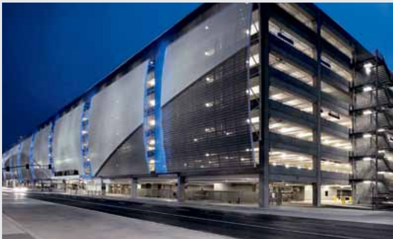
The eight-level structure contains 3,817 precast concrete components and is the largest precast concrete parking structure in the state of California, providing spaces for 3,350 cars.
