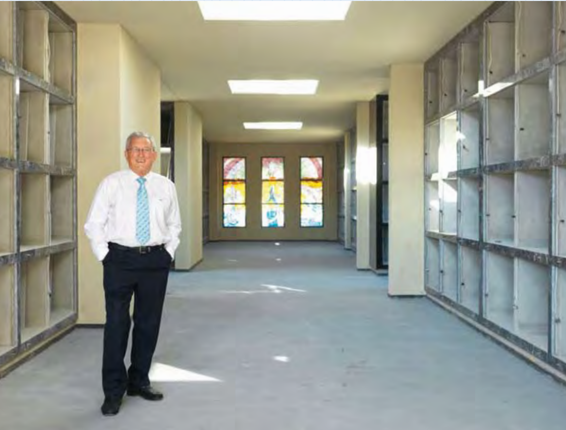
..... Ian Parker, Commercial Manager – Cemeteries and Crematoria, who manages many of InvoCare's major projects, at the construction of the new crypts at Pinegrove Memorial Park.
