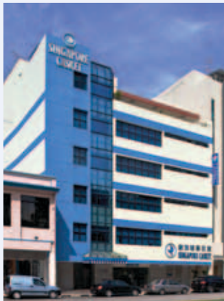
Top: Ann Wilson Funerals in Mon Vale, NSW. Right: The West Chapel at Rookwood Memorial Gardens and Crematorium in Sydney, NSW. Above: Singapore Casket Company's main Parlour complex and facility in Singapore.
