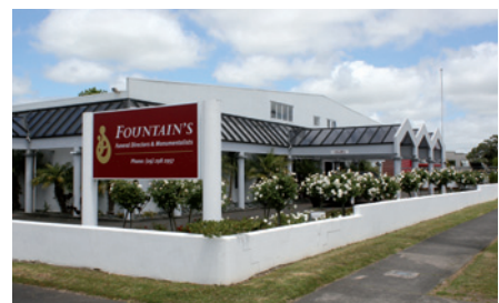
Fountain's Funeral Services in Papakura, Auckland, New Zealand which was refurbished in 2012.
