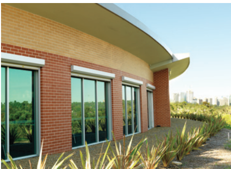
The new catering lounge at Northern Suburbs Memorial Gardens and Crematorium, Sydney which was built at a cost of over $7 million.
