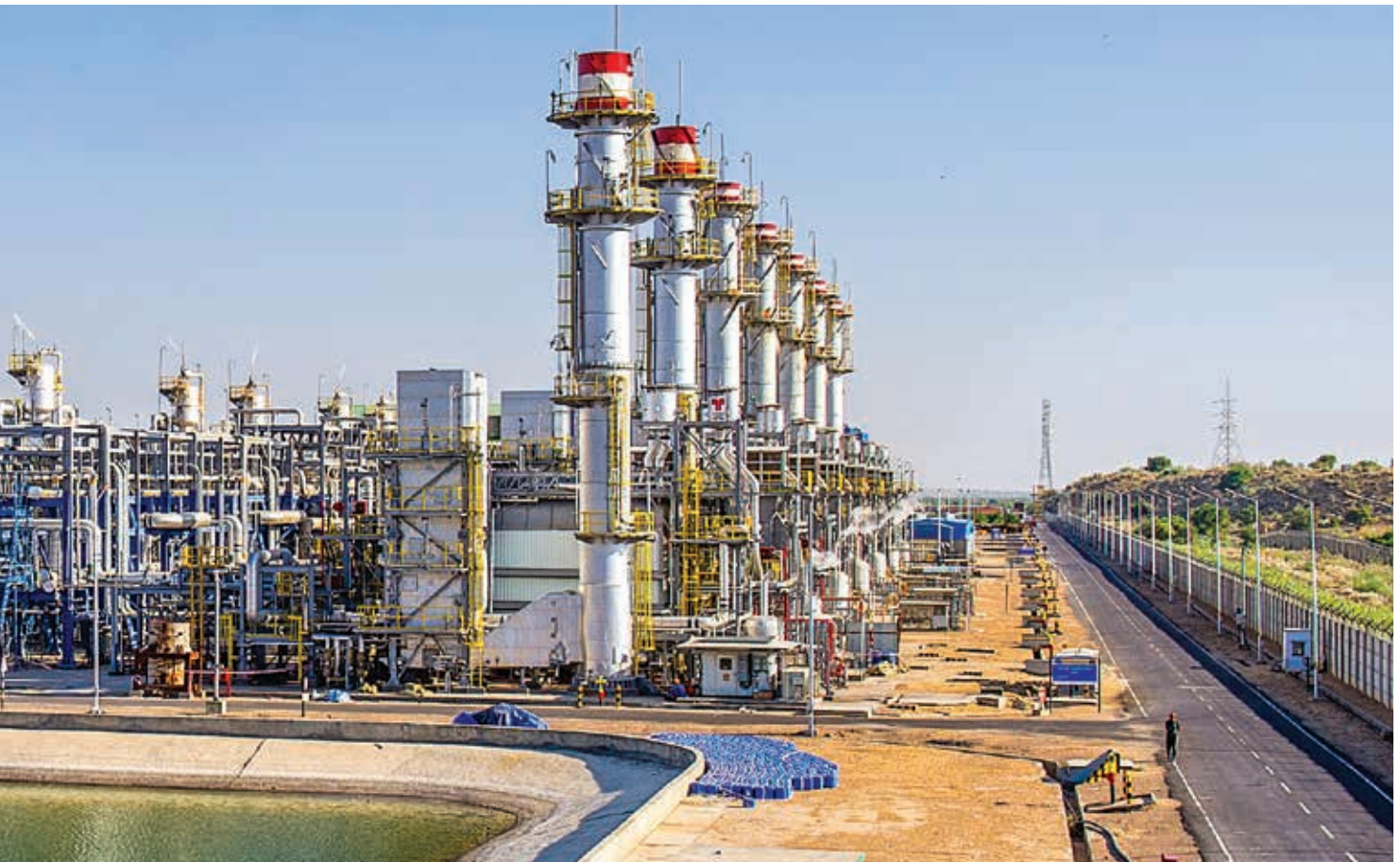
Mangala Processing Terminal, Barmer
