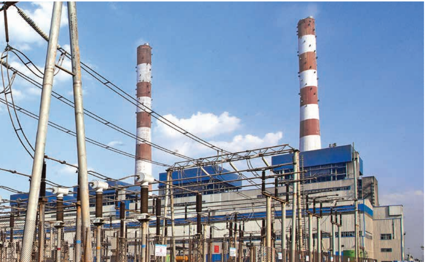
BALCO power plant
