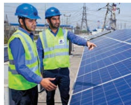
Solar panel installed in comprehensive building, BALCO
