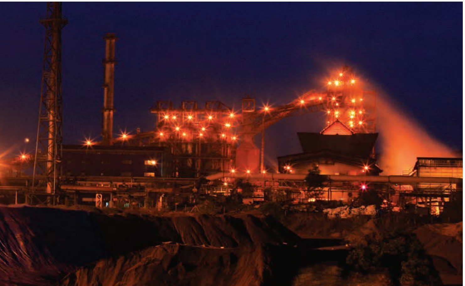
Pig iron plant, Amona, Goa
