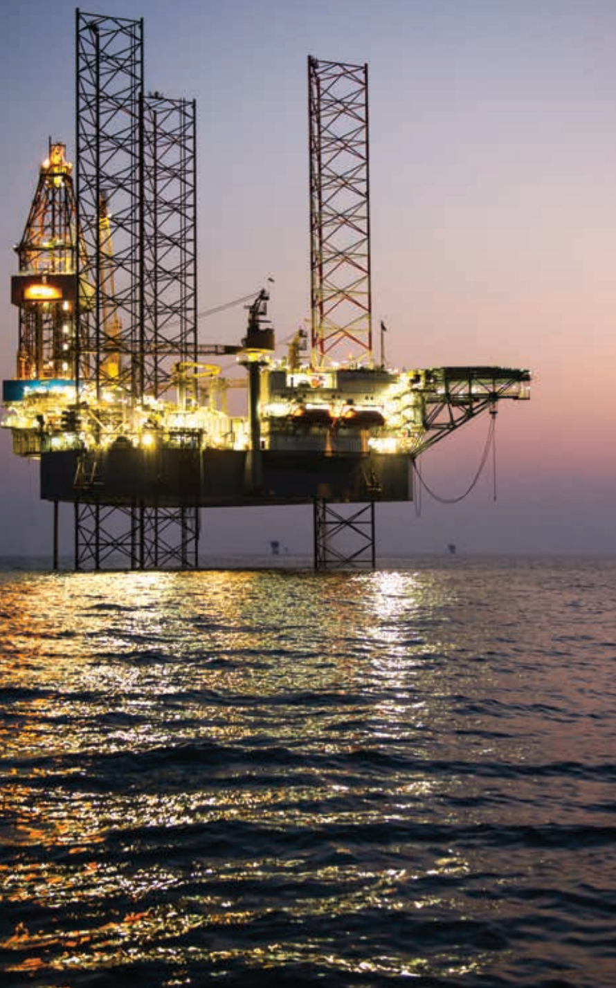
Offshore operations at Ravva
