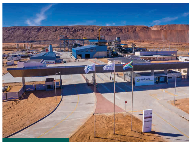
Zinc International Gamsberg Plant
