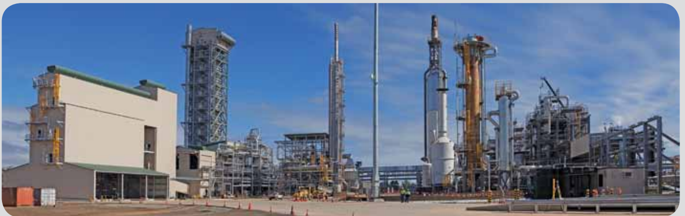
Moranbah ammonium nitrate plant
