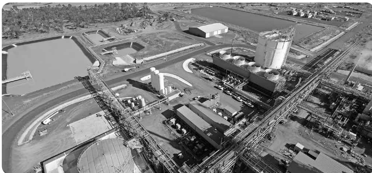
Moranbah ammonium nitrate plant.
