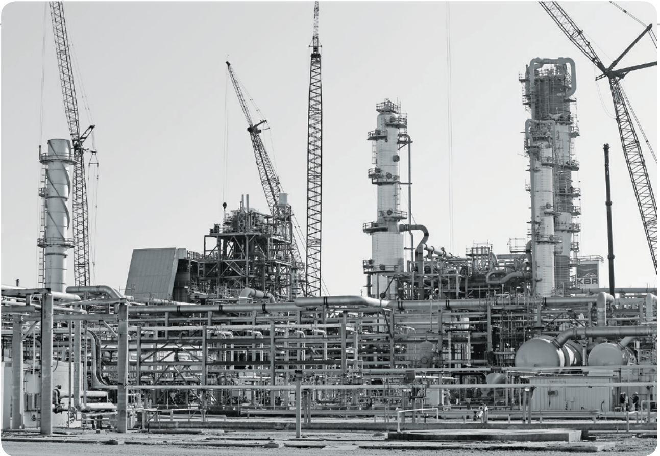
IPL Ammonia plant currently under construction at Waggaman, Louisiana.
