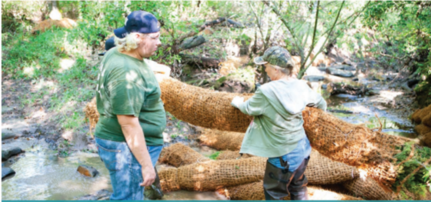
Partners working together installing coconut fiber rolls. Properly installed, these rolls prevent streambank erosion and help establish vegetative buffers. This improves water quality and habitat for aquatic life in the stream.
