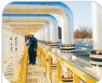
Construction of the Highland compressor station in Michigan has increased capacity of the Vector natural gas pipeline to 1 billion cubic feet per day.
