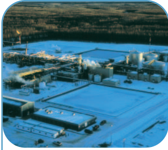
Bitumen production from MacKay River was connected to the Athabasca System in 2002.
