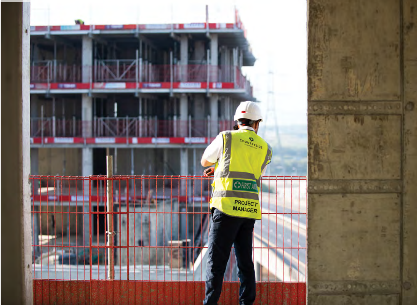
Fresh Wharf, Barking
