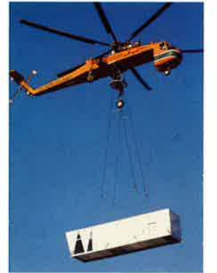
Installing 140 ton VAV rooftop unit.
