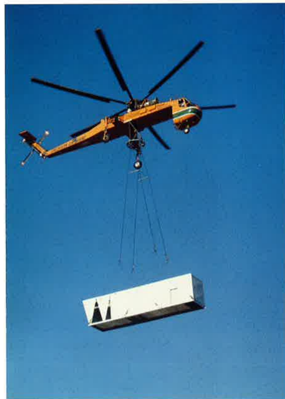
Installing 140 ton VAV rooftop unit.
