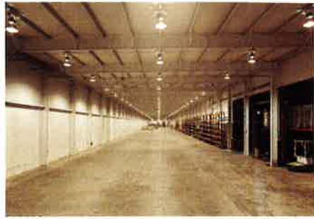
Future 25-60 ton assembly area.
