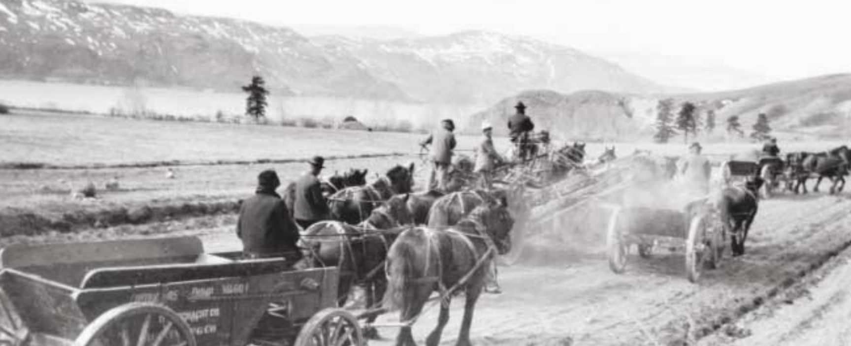
Horse-drawn equipment used to build railway roadbed; Tranquille, British Columbia, circa 1910
