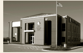
Iowa Savings Bank, Main Office
