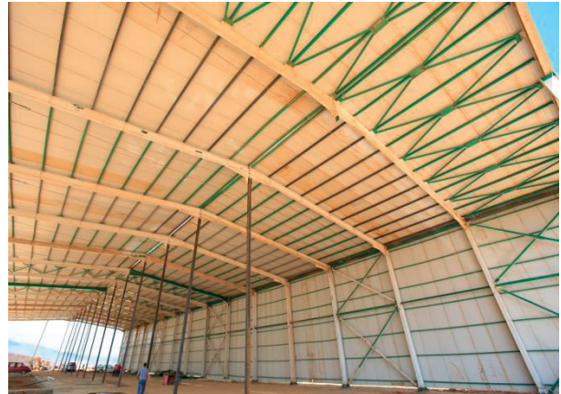
Figure 9 Internal panelling on the factory structure
