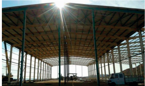
Figure 7 Factory under construction
