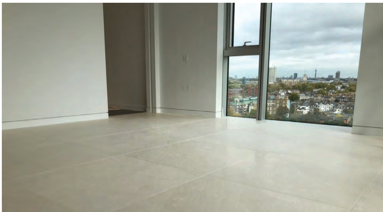
Figure 7 – Illirico Bianco flooring installed at Lillie Square
