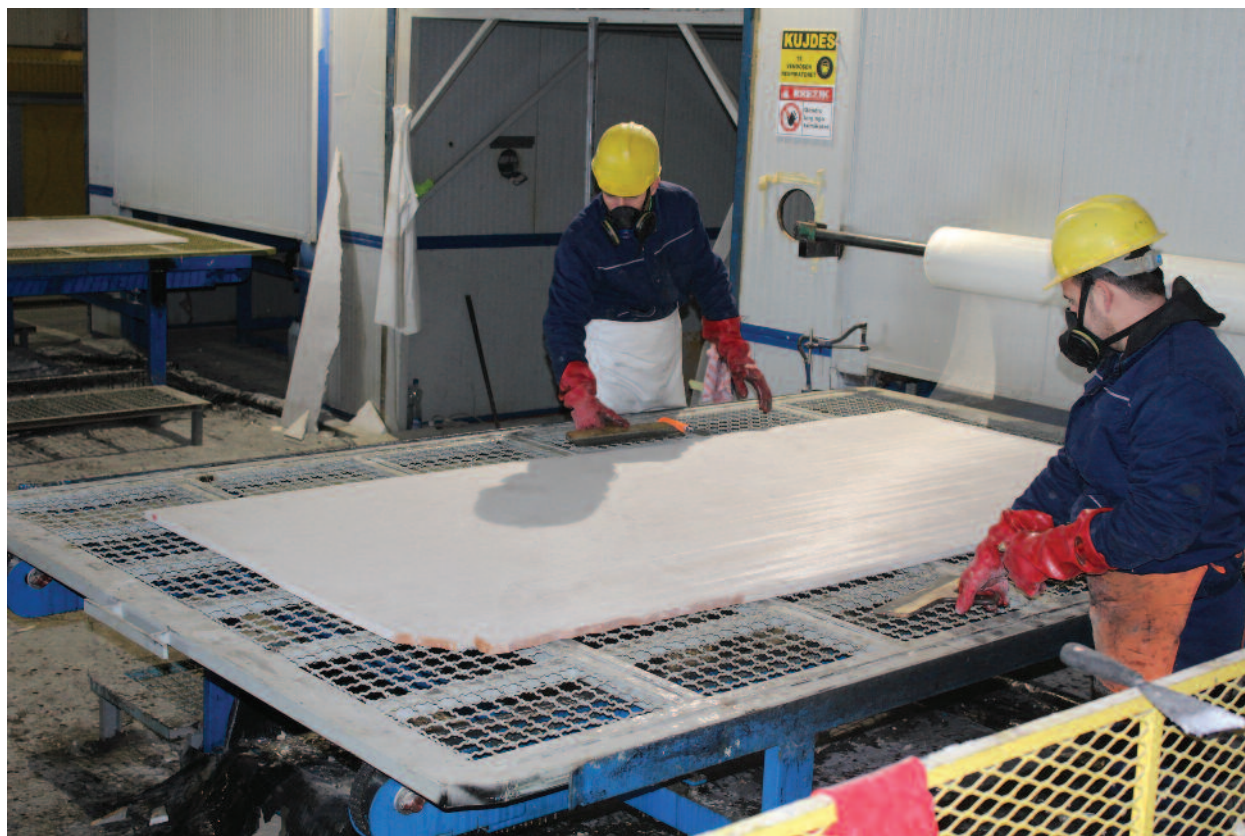
Figure 2 – Finishing work in the factory
