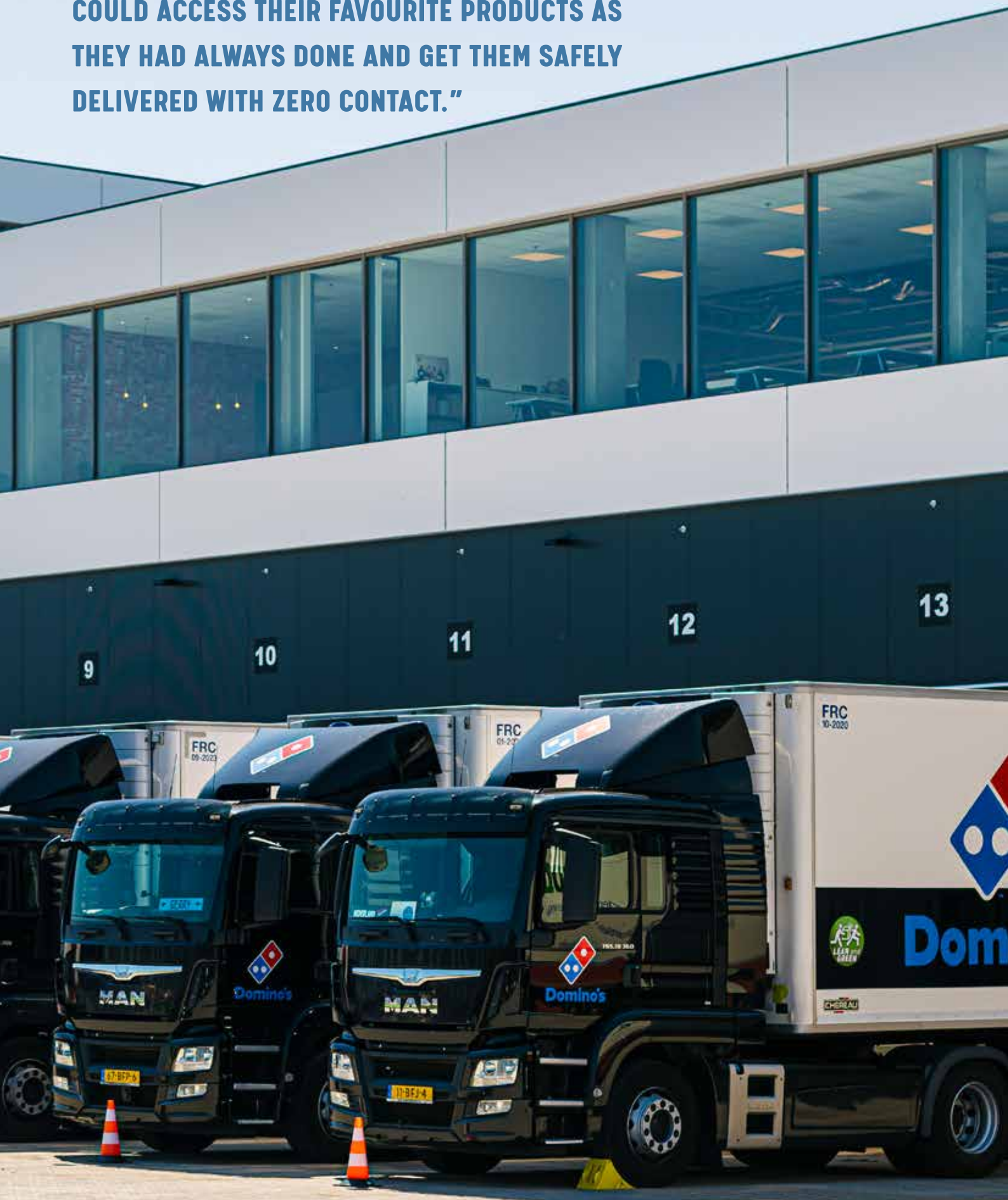
Supply trucks outside our new Nieuwegein Supply Chain Centre (Netherlands)
