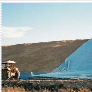
Wheat storage (under construction)
