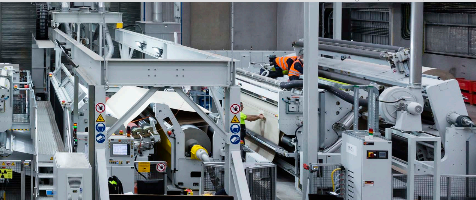
New state-of-the-art coating facility in Melbourne, Australia
