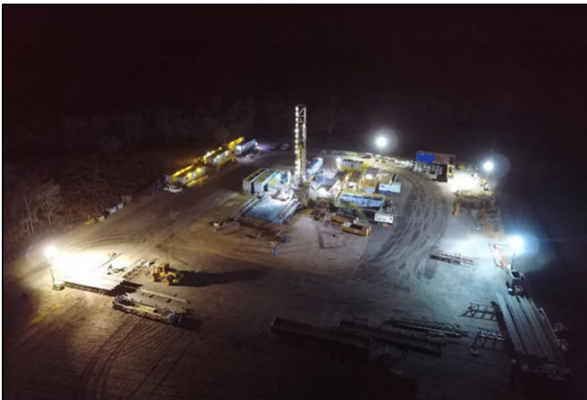
FIGURE 5 Myall Creek Well 4A
